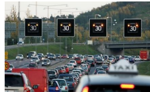
Motorway control systems
