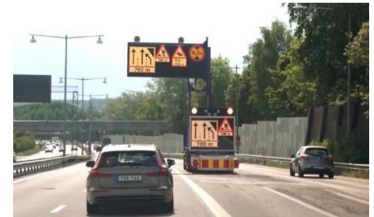
Road works warning
