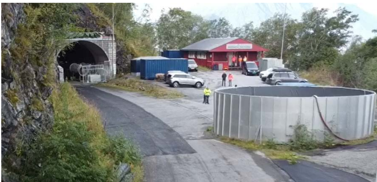
Oversikt Runehamar test tunnel
