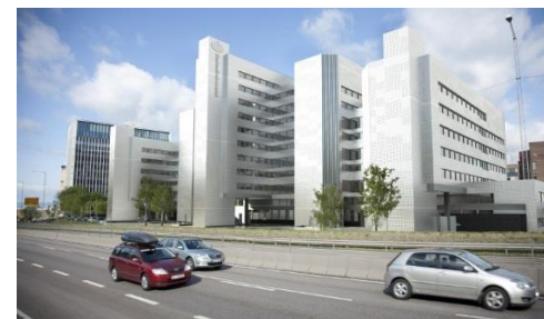
Fredrik Selmers vei 4, Oslo Skatteetaten
